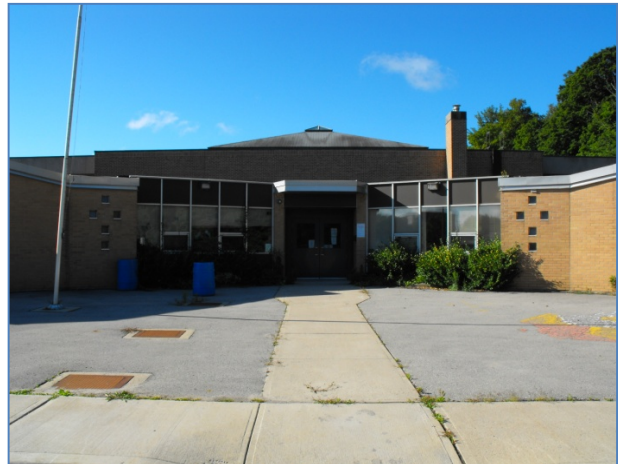
Figure 9 Former Holy Name School
